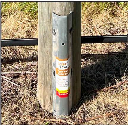
Ocloc half post repaired with Ocloc V
