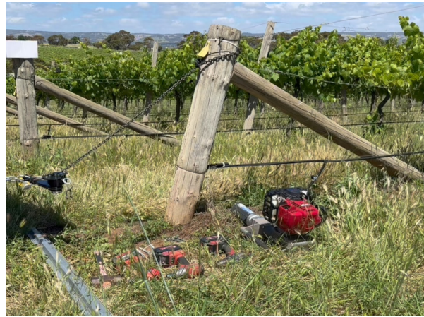
Using continuous chains /tractor to pull the broken strainer back onto the Ocloc SR.
