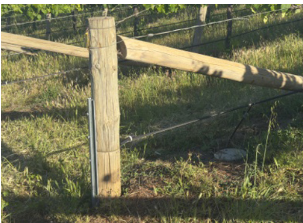
Strainer is repaired.
