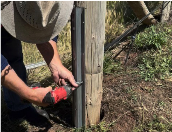
Drive in the shark tooth screws through the side slots starting at the bottom .
