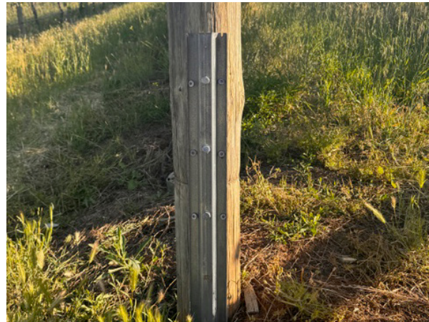
Drive in coach bolt screws in central holes with socket wrench.
