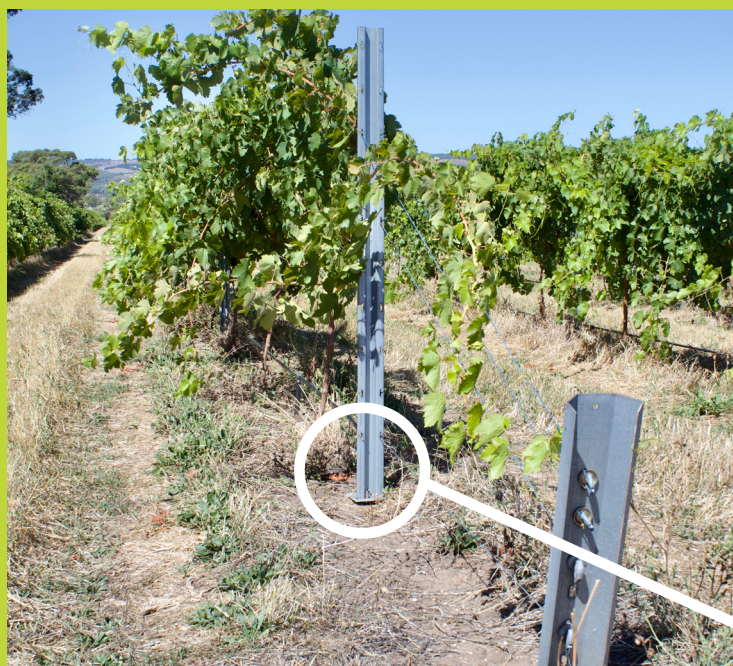
Anti sink plate: First in trellis post
