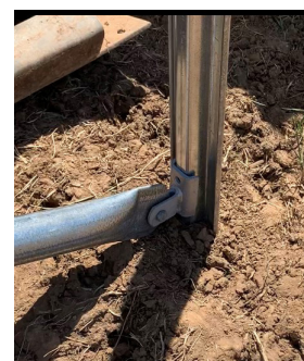
First in bracket attached to the angled stay via the pre-punched bolt hole in the A or W post
