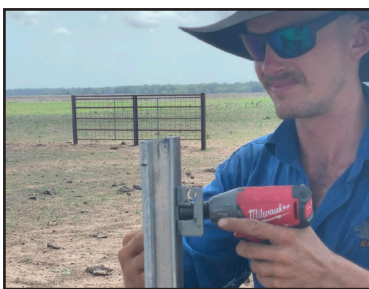
The OKBC and the RBC can be ratchet driven onto the post
