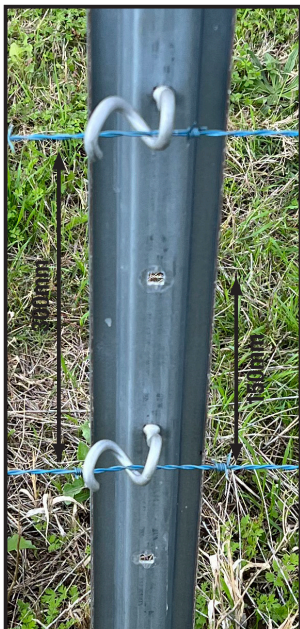
Placement of barb wire on post 150mm or 300mm options
