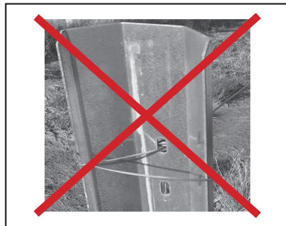
Example of incorrect attachment
