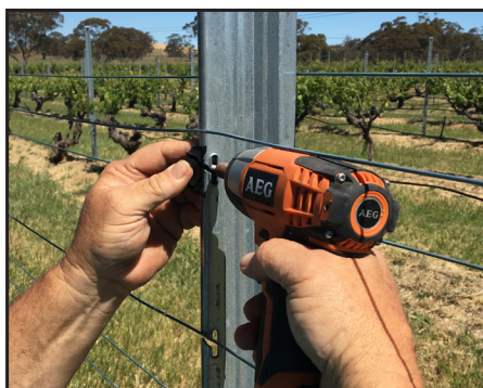
Ocloc 'K' clip being attached.
