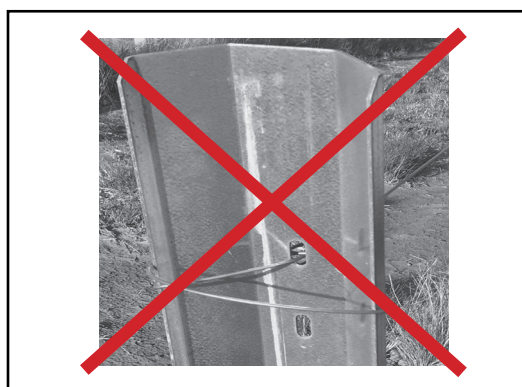
Example of incorrect attachment
