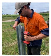
STEP 🕑 Secure the perch with bottom bolt and top bolt.
