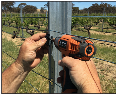
Ocloc 'K' clip being attached.
