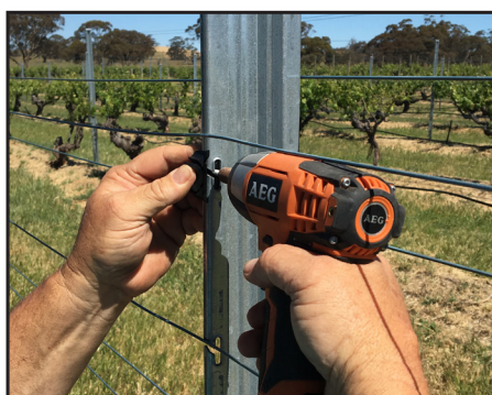
Ocloc 'K' clip being attached
